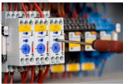
Electrical repairs are not capitalised as PP&E
