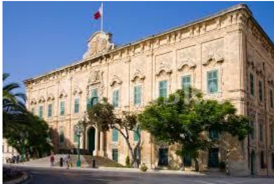
Auberge de Castille: operational heritage asset
