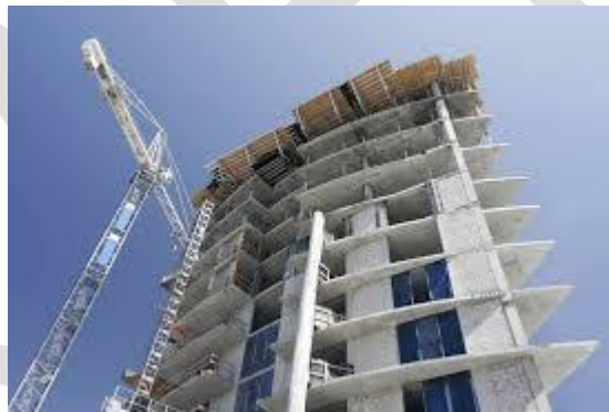
Building under construction
