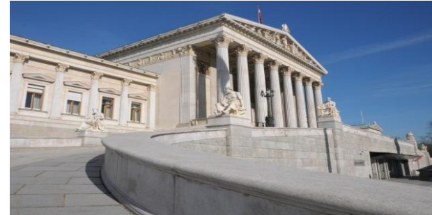
Historical Parliament Building - ramp area 33,89 Mio. EUR
